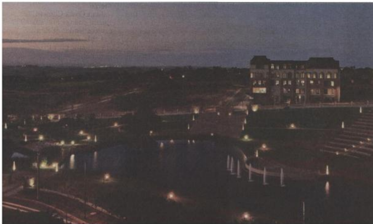
The Lincoln on Lake building overlooking Chris Saunders Park in uMhlanga Ridge. A multimillion-rand photovoltaic solar power system has been installed on its roof and the building is set to secure a Green Star rating from the Green Building Council of SA.
